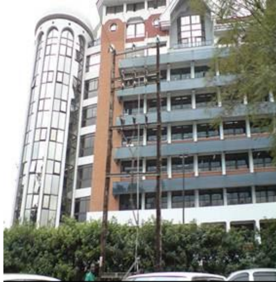
Plate 3: Britam office towers within the vicinity
