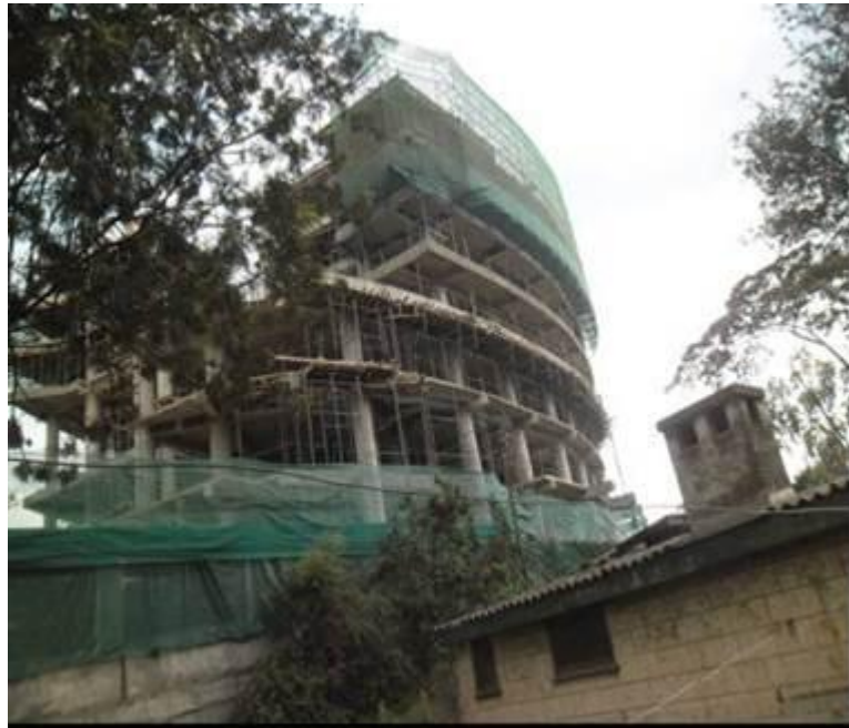
Plate 7: Mwalimu SACCO Ltd. Headquarters under construction next to the development plot
