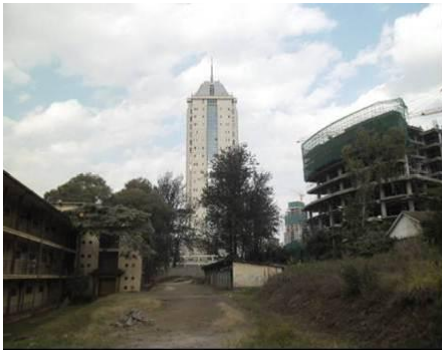
Plate 8: Rahimtulla Towers East of the proposed site
