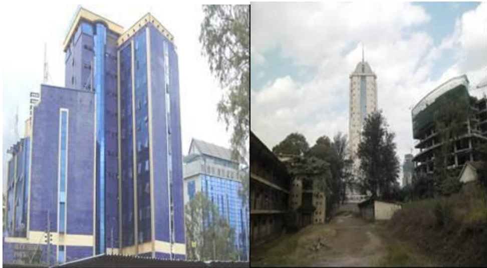
Plate 1:Blue Shield Towers and Rahimtulla Towers are office towers within the vicinity
